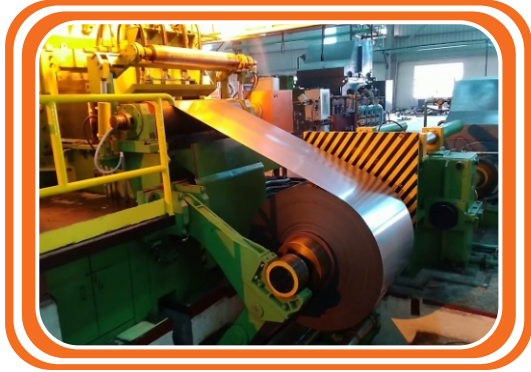
6 HI COLD ROLLING MILL
